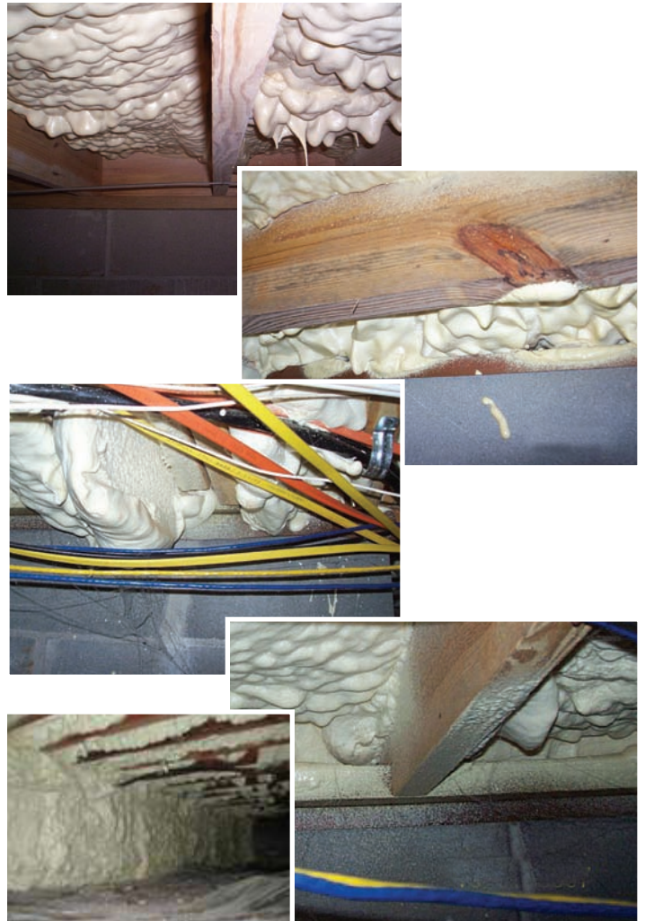
The photos below were taken in the house above. You can see how the foam insulation covers much of the wooden members under the crawl space, making it impossible to inspect for termite activity above the foam. Termites burrow into the foam in search of viable wood.
